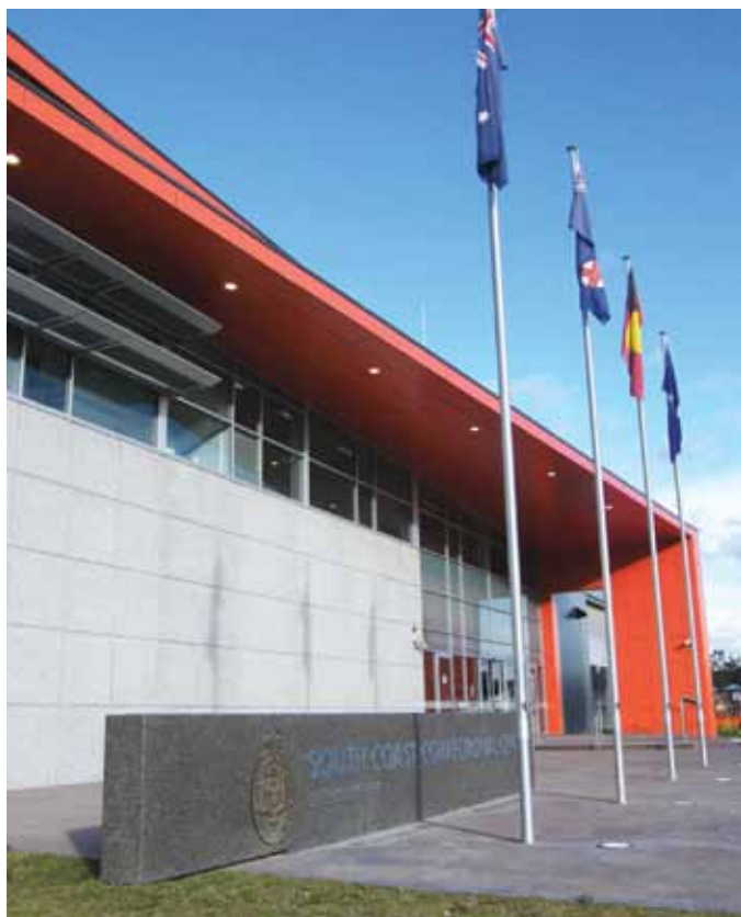
The South Coast Correctional Centre – officially opened in November 2010
